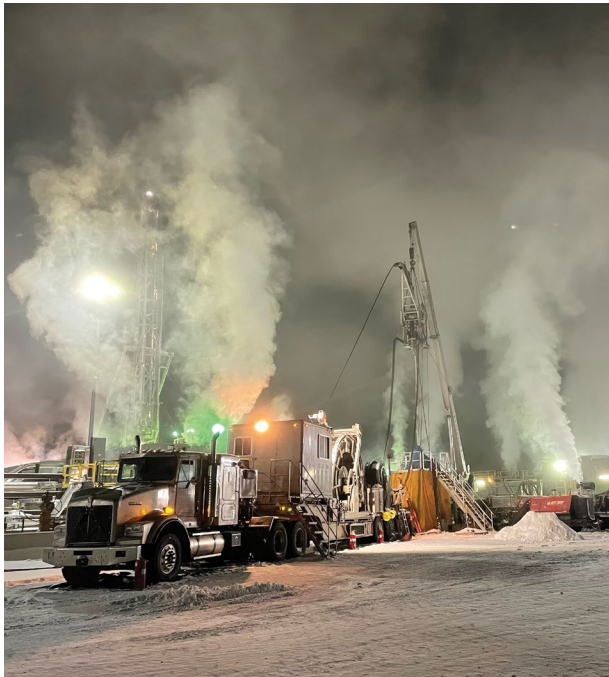
Photo by Rustem Sharifullin Foster Creek job operating at -40°C
