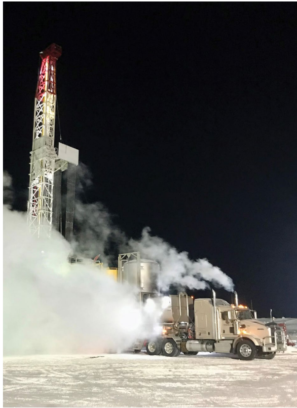
Photo by Ty McKernon -Twin Cementer Pumping in -45°C
