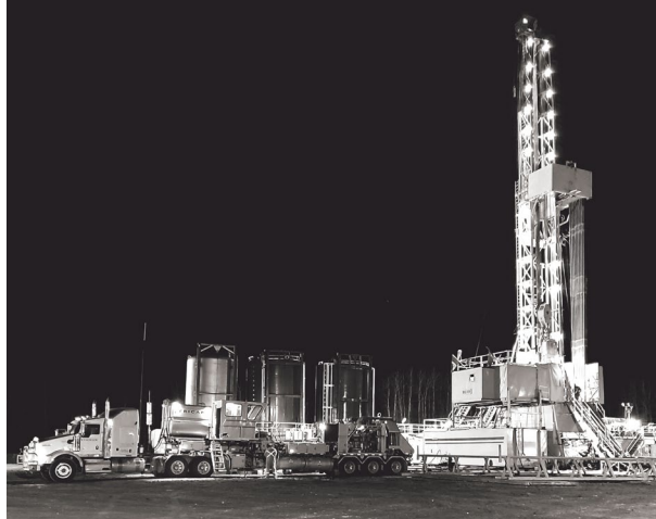
Photo by Rob Moulton - Surface Cement Job
