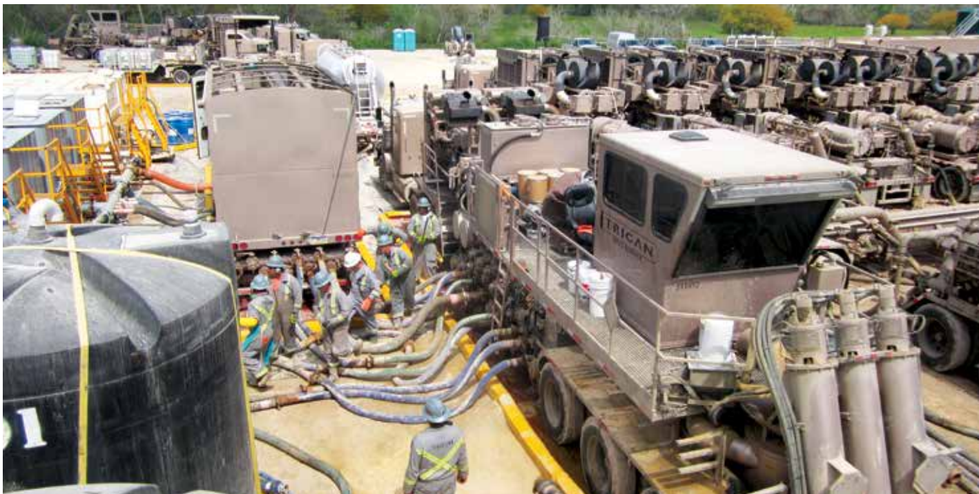
Frac blender and pumps after rig up.
